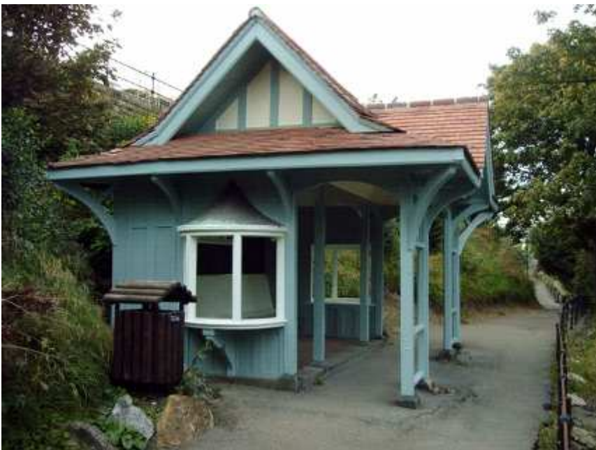
Repaired Shelter pictured September 2007
